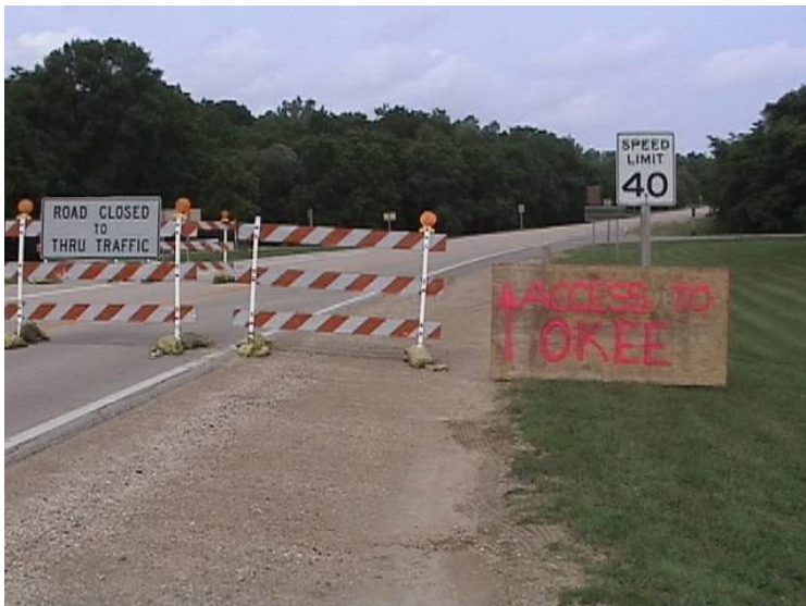
OK, temporary , but color is hard to read and will fade. Should be replaced with professionally made sign
